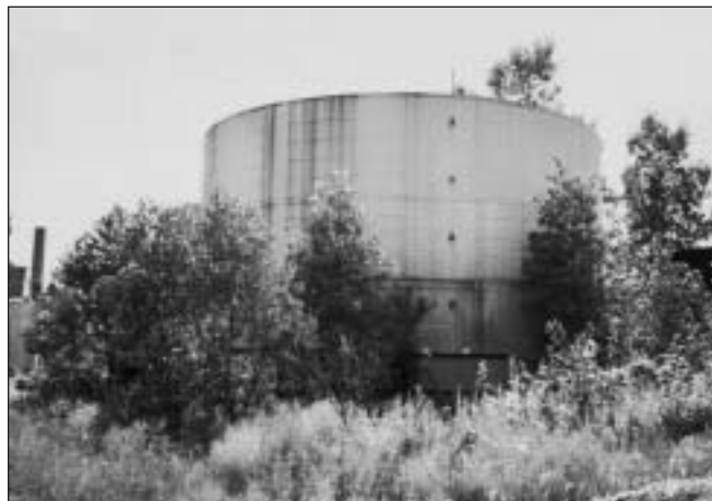
Adequate exterior inspection must not be hindered by excessive vegetation around a tank (Fig. 2).
