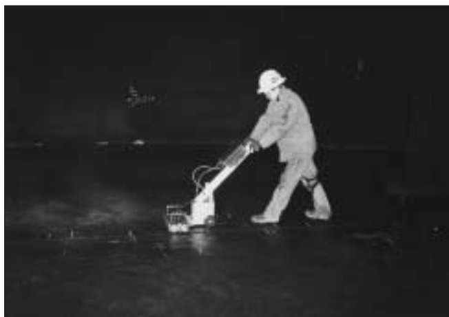
A qualified operator runs an MFE device over a tank bottom (Fig. 4).
